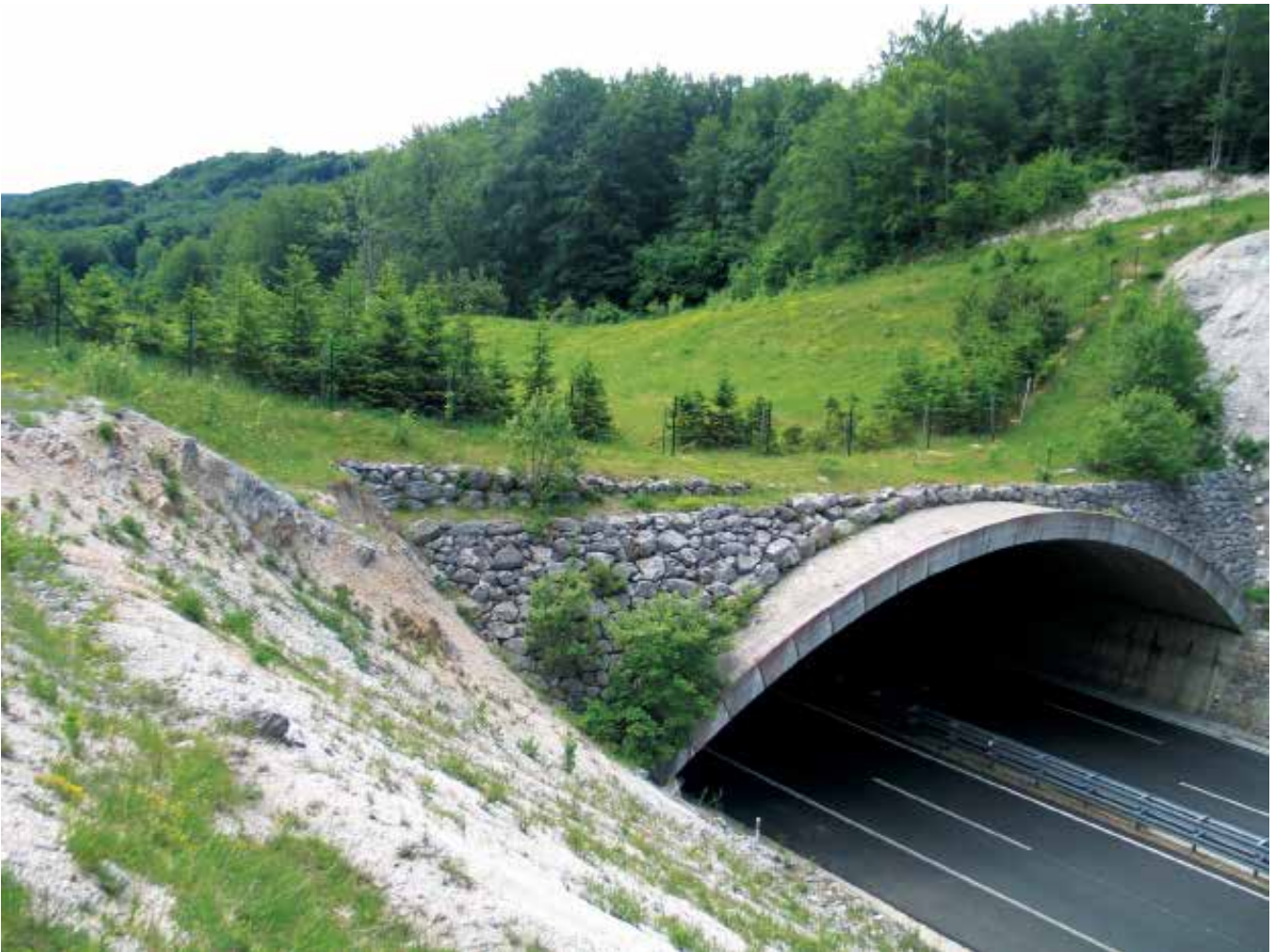
Wildlife crossing structures such as this highway overpass in Croatia, one of 13 in the country, are no substitute for an intact landscape but have value in mitigating the effects of fragmentation for many species. © Djuro Huber
